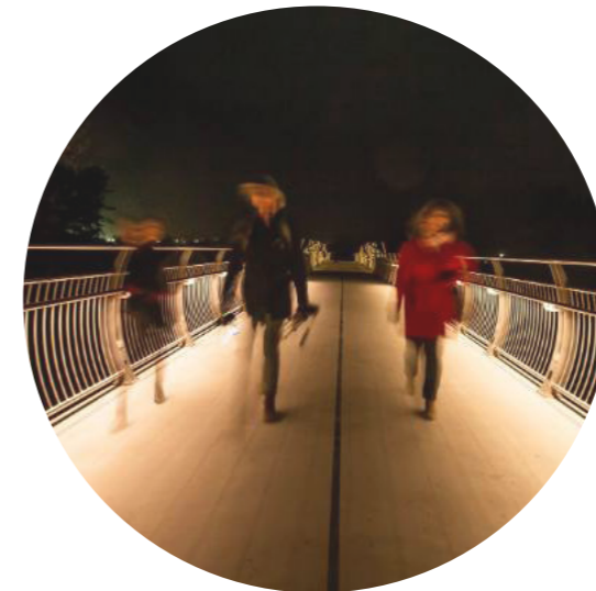
Example of the use of lighting on a bridge integrated into the handrails
